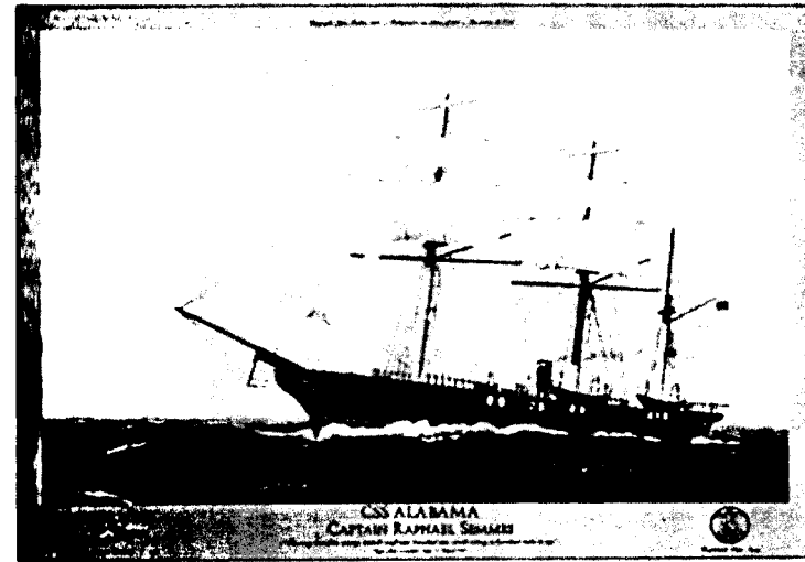
C.S.S. Alabama (cruiser), built by Laird, 220' x 31.9' x 14' at 1,050 tons;
