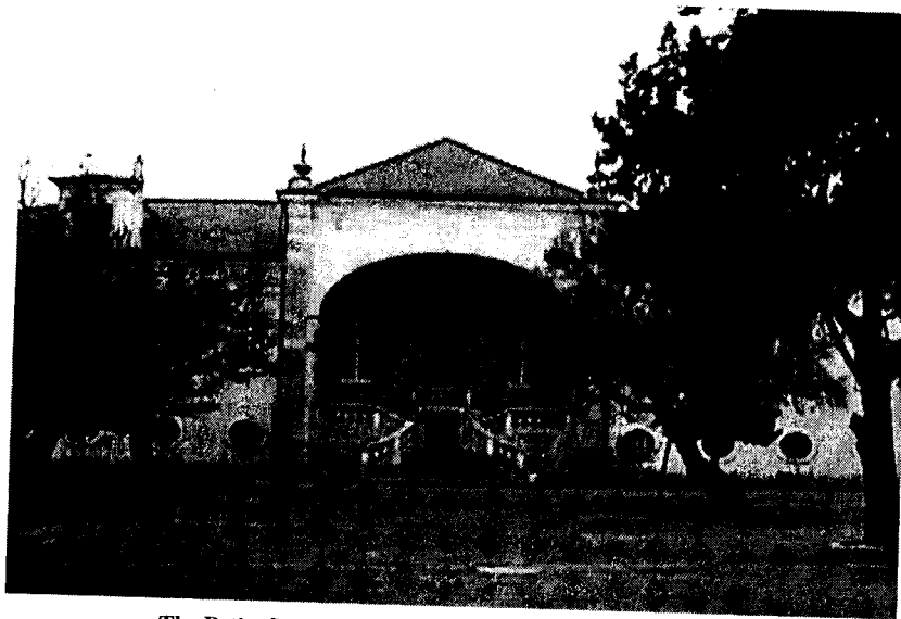
The Patio, St Julian's School (courtesy of Ormond Fannon)
