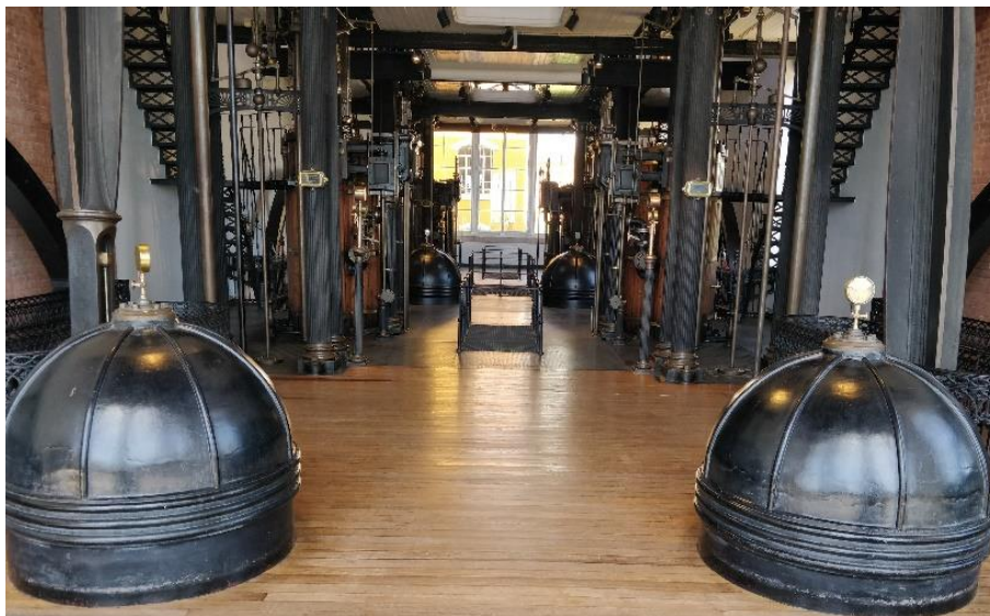
The Steam Engine Room
