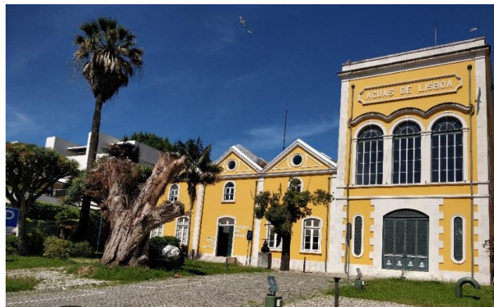
The Barbadinhos Pumping Station
