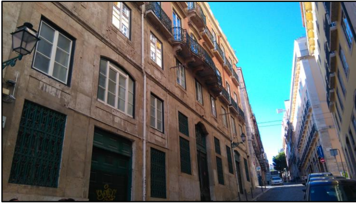
De Visme's townhouse on Rua das Flores, Lisbon
