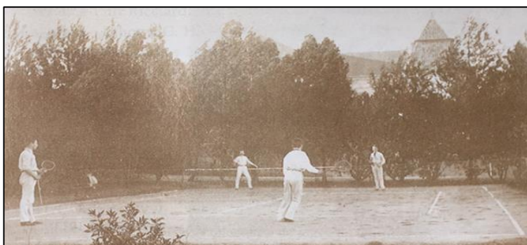
The tennis court at the Carcavelos cable station
